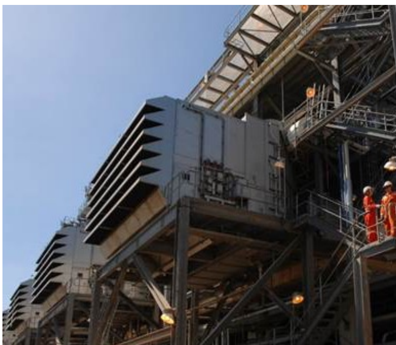
At the LNG plant, 720 pairs of Donaldson filters provide clean air to six LM2500 G4 gas turbines
